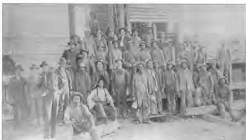
Work crew at No. 7 Shaft, Union Copper Mine
