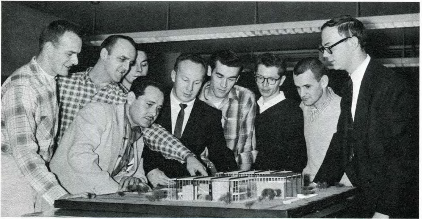
Mr. Noetzel answering Krupinski's question of a possible problem in the construction of this project.
