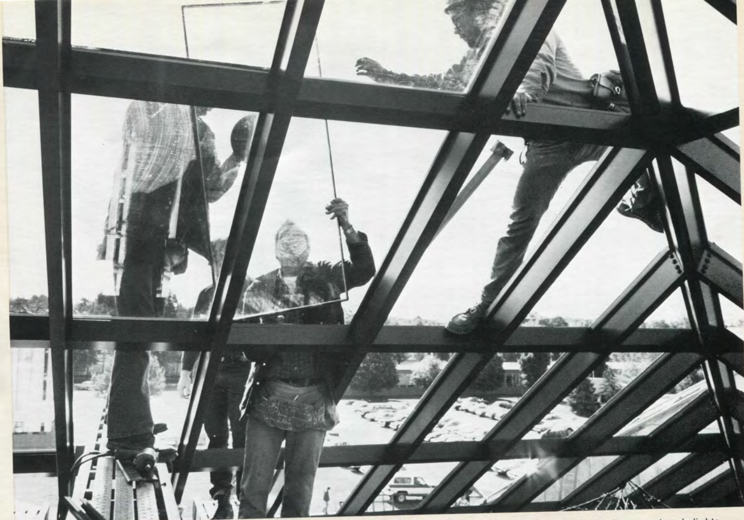
High above the campus, in September, 1981, glaziers carefully placed glass panels into the new Management Building's four massive skylights which will illuminate the structure's interior. To help reduce lighting costs, much of the building has been designed to take advantage of "free" natural light.
