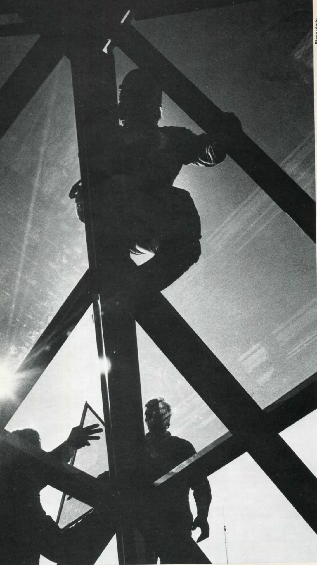
Piece by piece, glass panels in the Management Building's skylights are placed high over the central courtyard.
