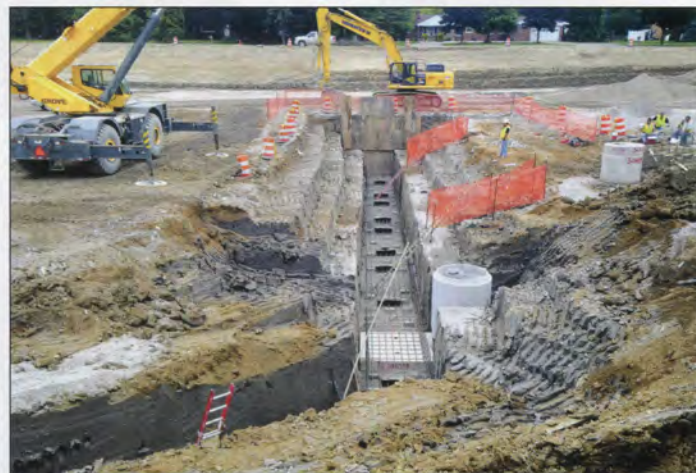
During the 167-day reconstruction project, MDOT constructed this 48-inch prestressed concrete water main under I-96, just west of Middlebelt Road in Livonia, for anticipated future use.
