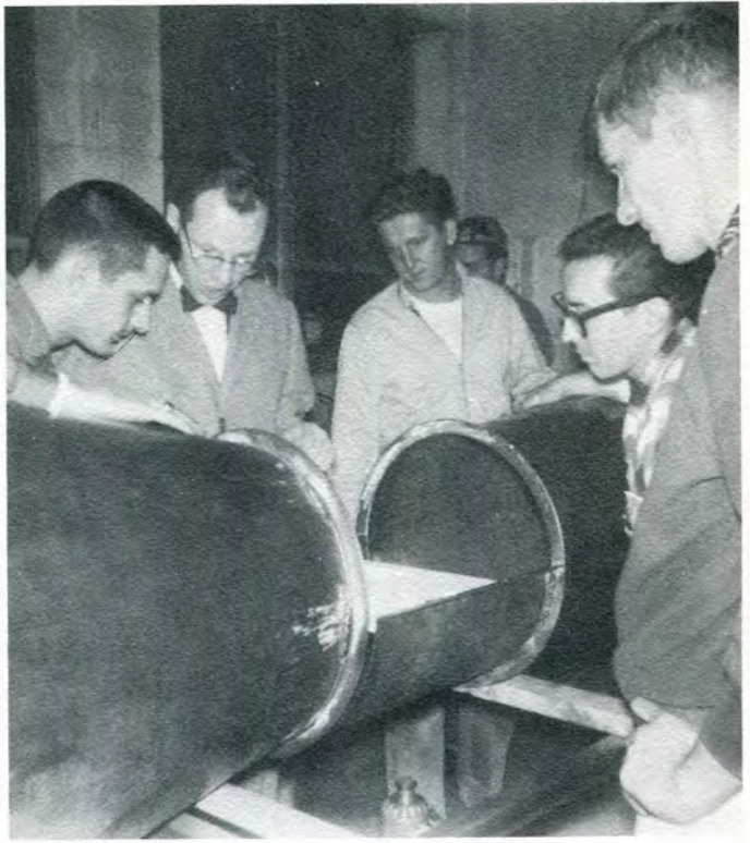
Phil Mendola, Professor Chambers, Harry Campion, Haider Belbeisi, Ross Vorpapel, and Bill Mooney, install the instrumentation platform in the S.A.E. wind tunnel.
