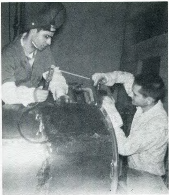
Haider Belbeisi and Phil Mendola weld supporting hoops on the S.A.E. wind tunnel.
