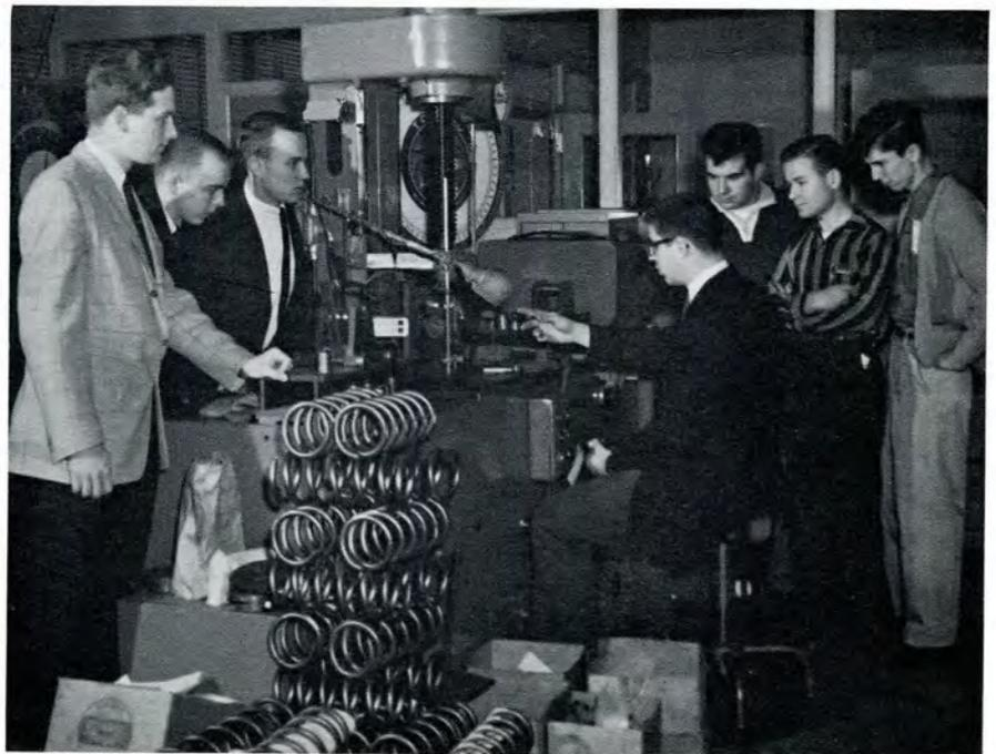
The members look on as one of the guides explains the method used to check the load limit of coil spring.
