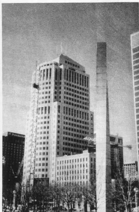
Figure 38 150 West Jefferson Building, Heller and Leake (1989).
