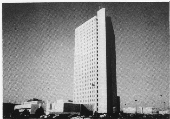
Figure 29 Top of Troy Building, Rossetti Associates (1976).
