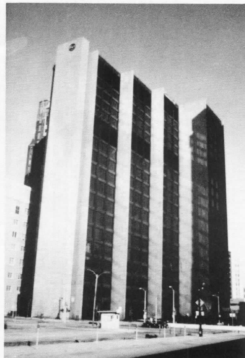
Figure 32 Michigan Bell Building, Smith, Hinchman and Grylls (1973).
