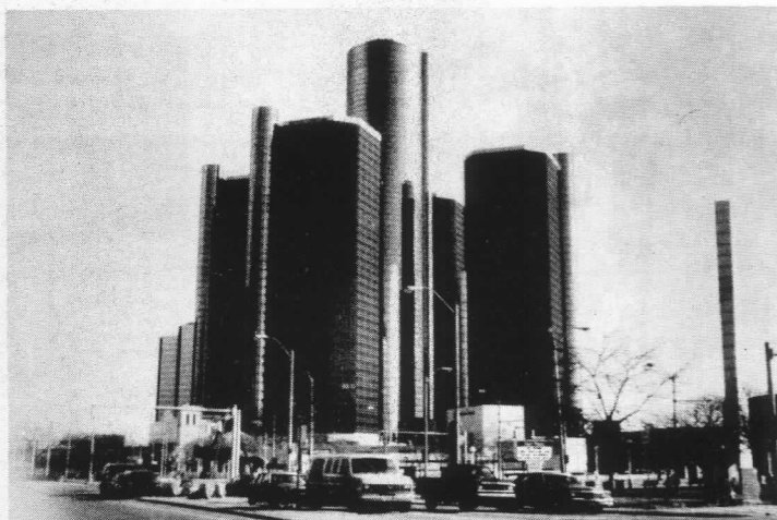
Figure 35 Renaissance Center, John Portman (1977).
