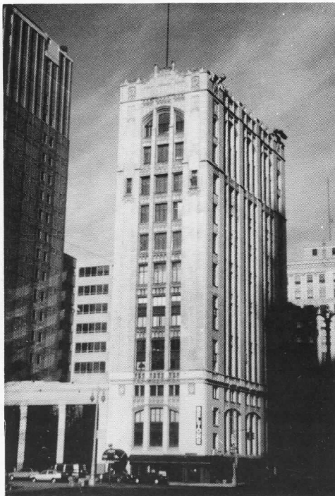
Figure 13 Fyfe Building, Smith, Hinchman and Grylls (1919).
