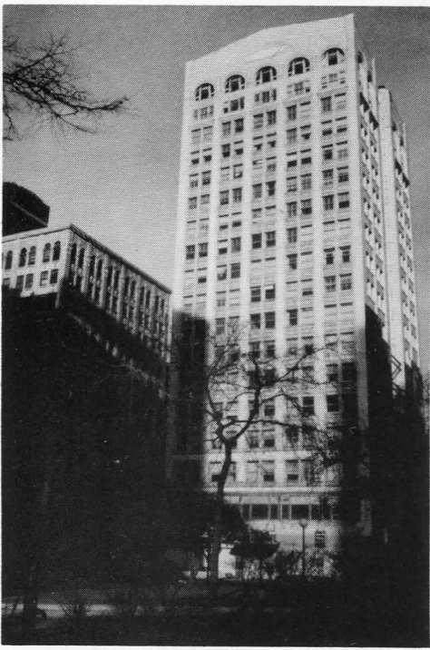
Figure 17 Kales Building, Albert Kahn (1914).
