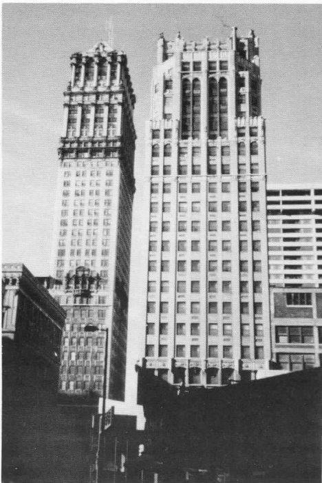
Figure 8 Book Tower (1926), Industrial Arts Building (1924), Louis Kamper.
