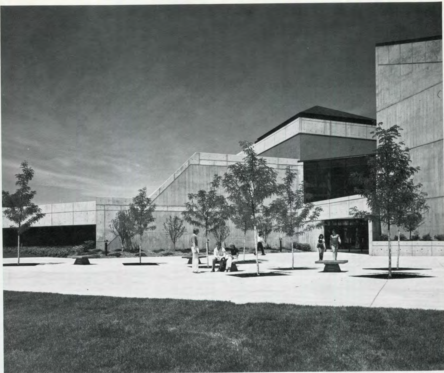
LIT's Wayne H. Buell Building, dedicated in May, 1982, houses the School of Management and the College library, dining room, bookstore, and several administrative offices.
