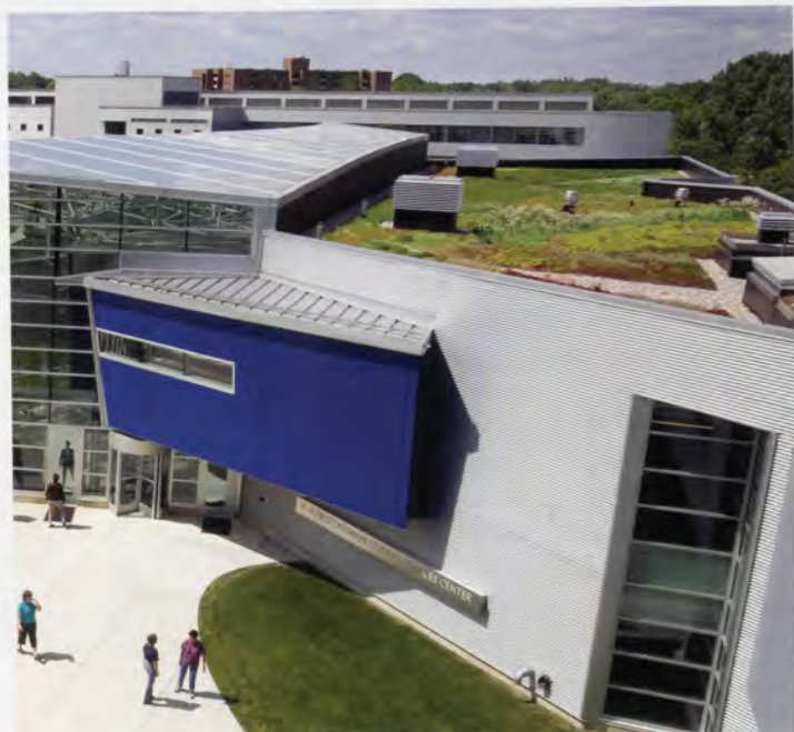
More than 60 percent of rain water is absorbed by the plants on the Taubman Center's green roof, and the remaining runoff is used as non-potable water in the building. Excess water is filtered through the quadrangle's bioswale before entering a Rouge River tributary cleaner than when it fell from the sky.
