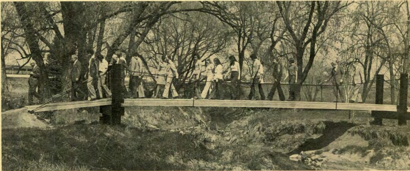
L.I.T.'s new student-designed footbridge over the Rouge River links the College's outdoor athletic facilities with the rest of the 85-acre campus.
