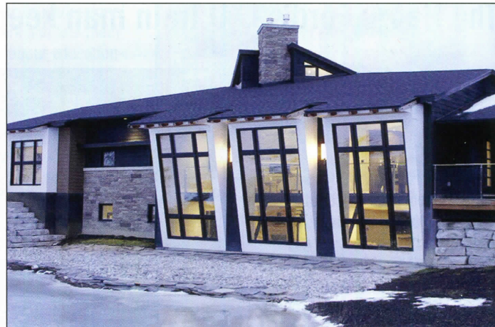
The south facade of the Delta House, showing the "Three Sisters" passive solar windows.
