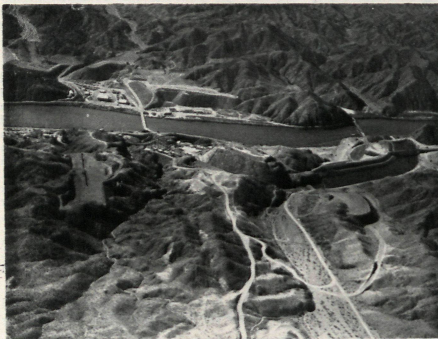
Bird's eye view of the site of the new Davis Dam. The dam proper will be built between the two bridges which can be seen crossing the river in this picture.
