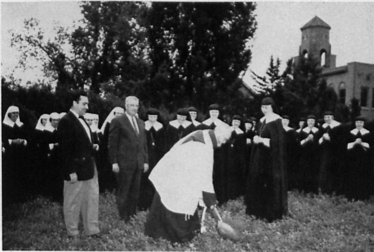
Father Thomas Aquinas, after blessing the site, tries his hand at the shovel. At the left of Father are Mr. James McCarron, Fort Wayne, architect; and Mr. Donald Norwood, Huntington, general contractor.
