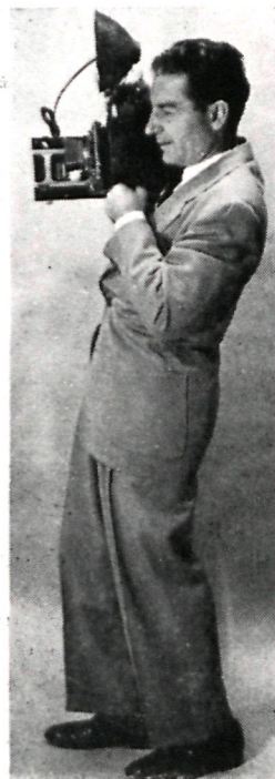
This is going to be a good one.
