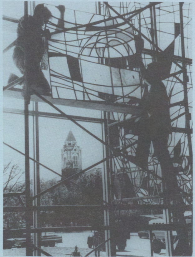
Installation of the Burning Bush window, October 1967.
