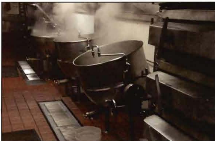
Before (top) and after (bottom) pictures of the renovations done in the Dining Hall kitchen.
