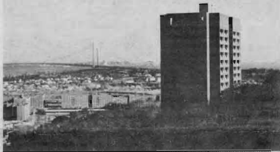
Now housing 372 students, Harbor View is again nearing capacity.
