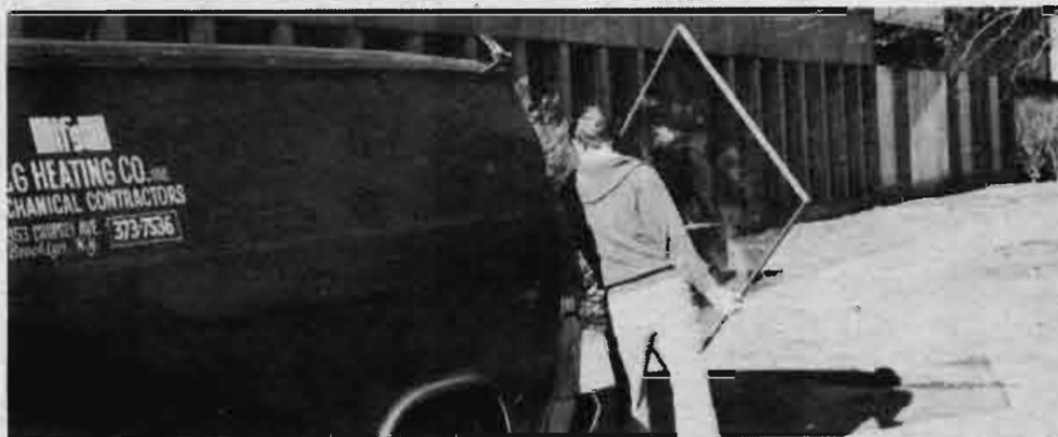
Maintenance man restoring the science hall back to normal.
