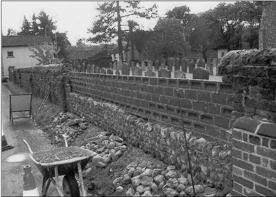
Wall repair at Shipdham's All Saints Church
