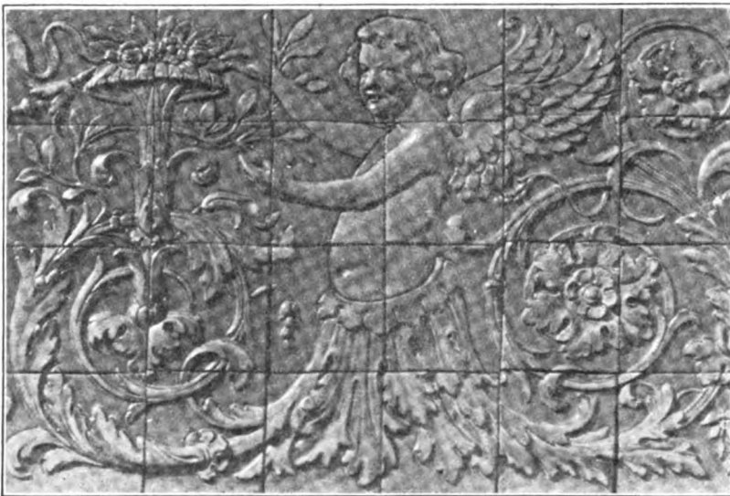
Faience Frieze Exterior School House, Newark, N. J.
