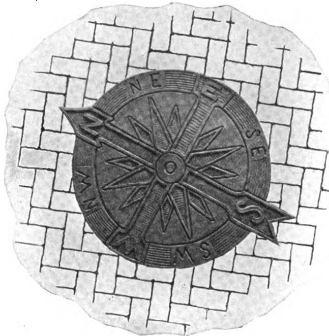
Compass in Clay Tile Set in Brick Pavement.
