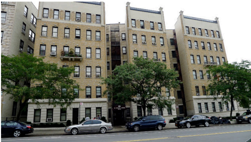
928-930 St. Nicholas Avenue, the "Historic Hall" Apartment Building
