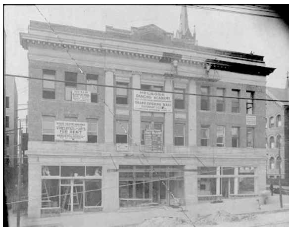
"The facade of the Bronx Theatre under construction" by the Byron Company (New York, NY). From the Collections of the Museum of the City of New York; http://collections.mcny.org/C.aspx?VP3=SearchResult_VPage&VBID=24UP1G75YD08&SMLS=1&RW=1276&RH=664
