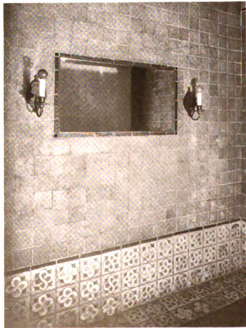
BATHROOM. BASE OF PERSIAN TILE, WALLS OF UNGLAZED BISCUIT TILE. AETCO BUILDING THE NEW YORK OFFICES OF THE AMERICAN ENCAUSTIC TILING CO.
