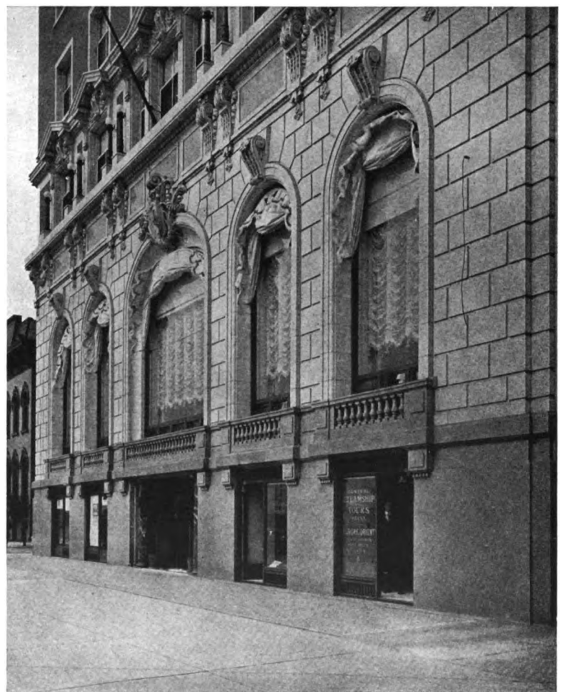
Detail of Lower Stories on Michigan Boulevard
