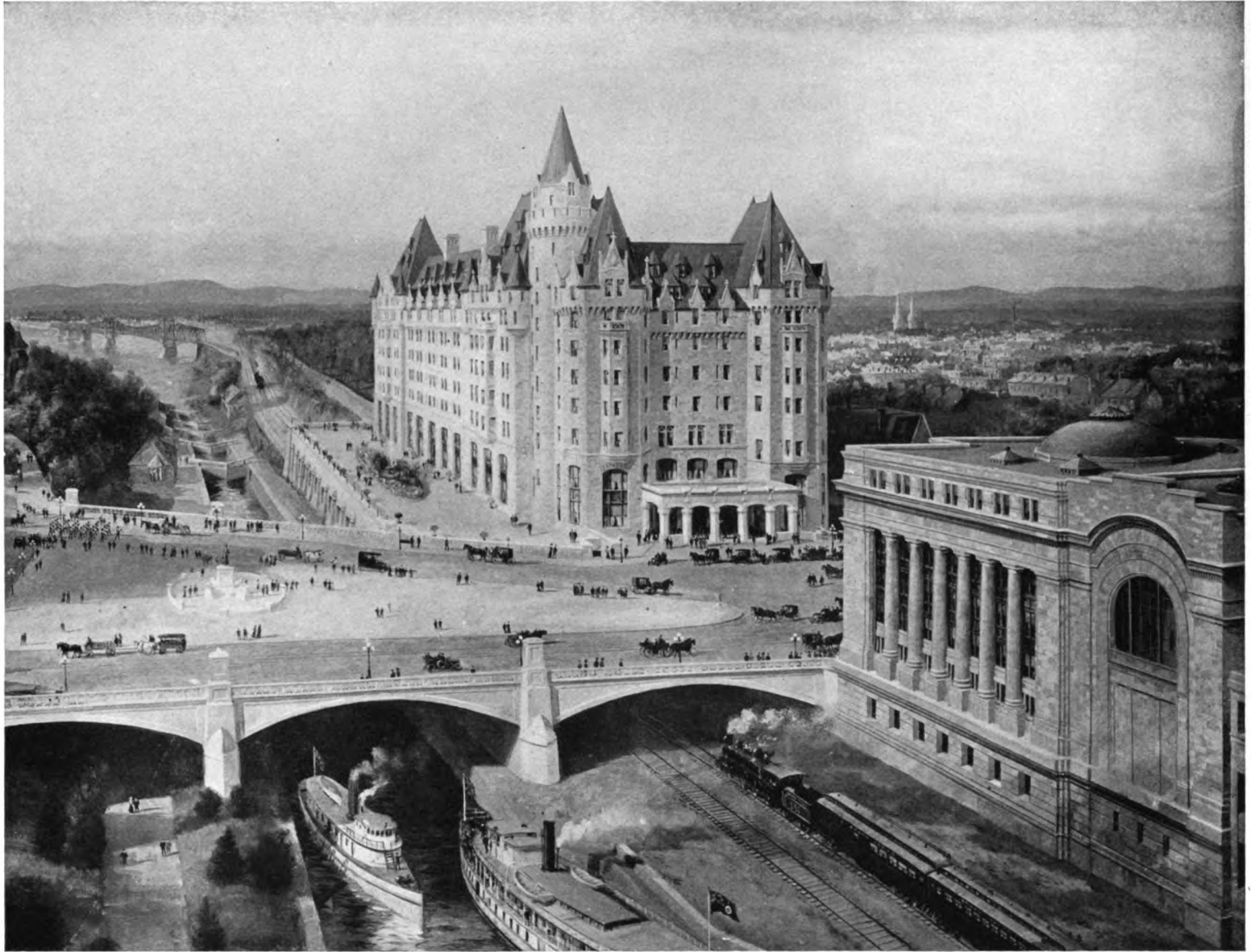
General View, Showing Relation of Hotel to Railroad Terminal
