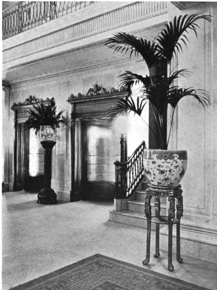
Detail of Entrance Doors in Lobby
