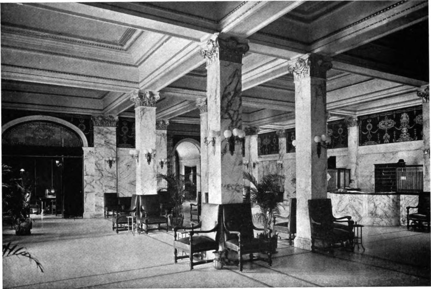
View in Lobby
