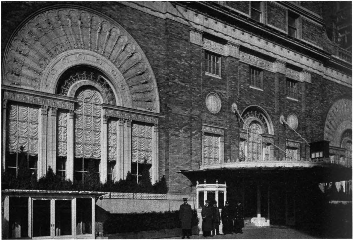
Detail of Lower Stories of Park Avenue Façade
