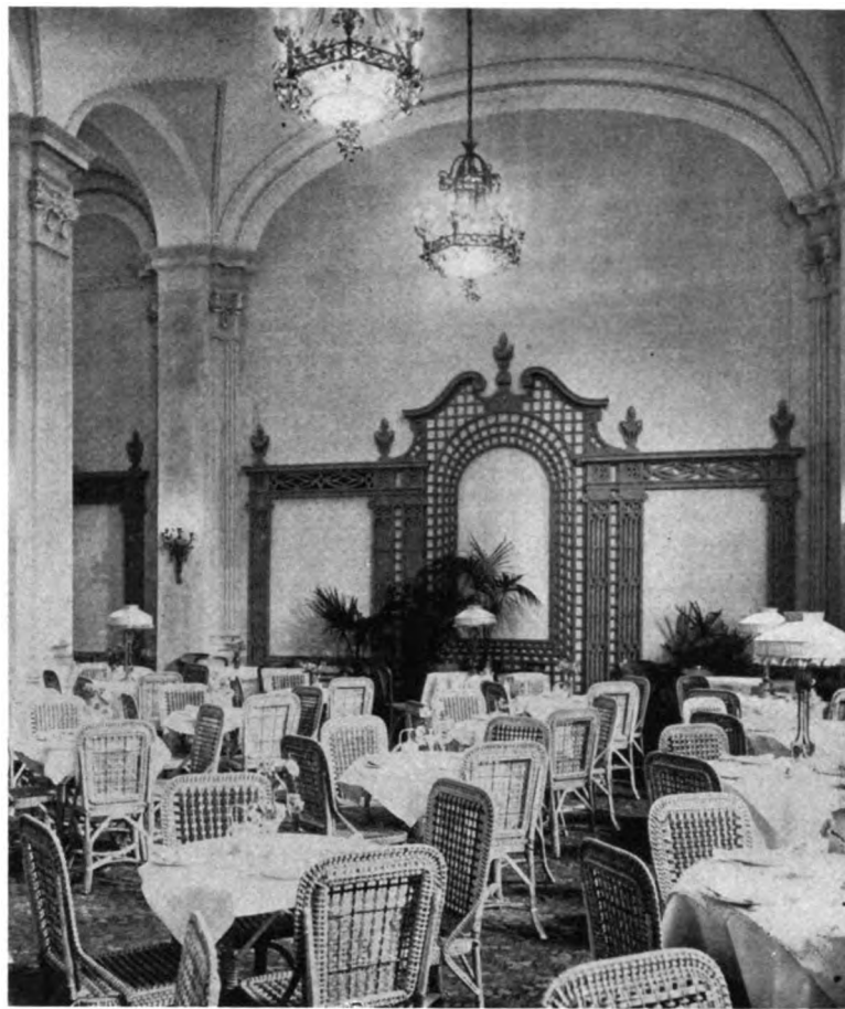
The Palm Room is finished in imitation Caen stone, with a vaulted ceiling. The lattice-work and the Canton furniture add a refreshing note
