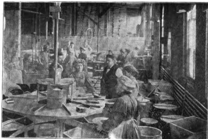
TILE MAKING AND PRESSING ROOM.
