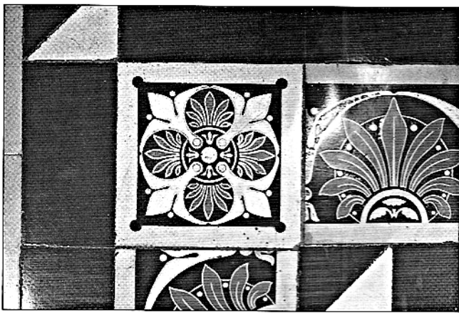
Figure 5 The encaustic tiles that surround the geometric tiles at the heart of the centrepiece on the ground floor.
