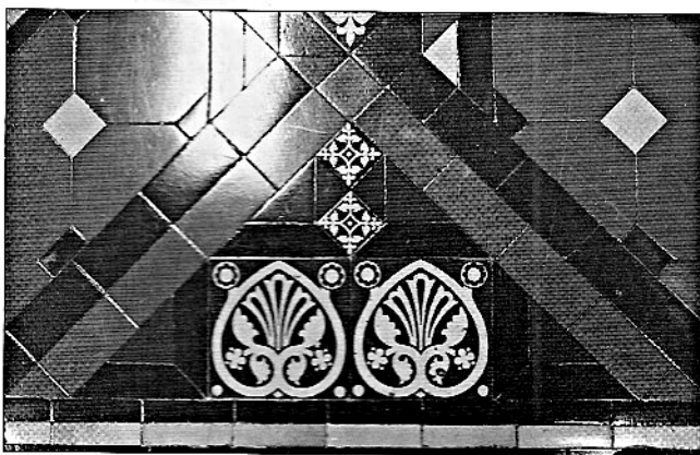
Figure 6 Some of the encaustic tiles that form part of the centrepiece on the ground floor. The largest ones measure 6 inches by 6 inches
