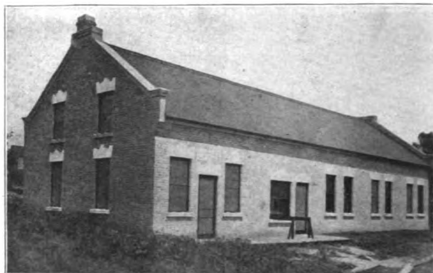
THE NEW BRICK OFFICE BUILDING.
