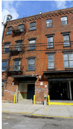
98 West Street, Greenpoint. This building and the building that held Charles Volkmar's pottery connected via internal passageways. They may have opened to a common field-type area in the backs of the buildings in the 19th century where the kilns were probably situated. (Photo courtesy of Michael Padwee)
