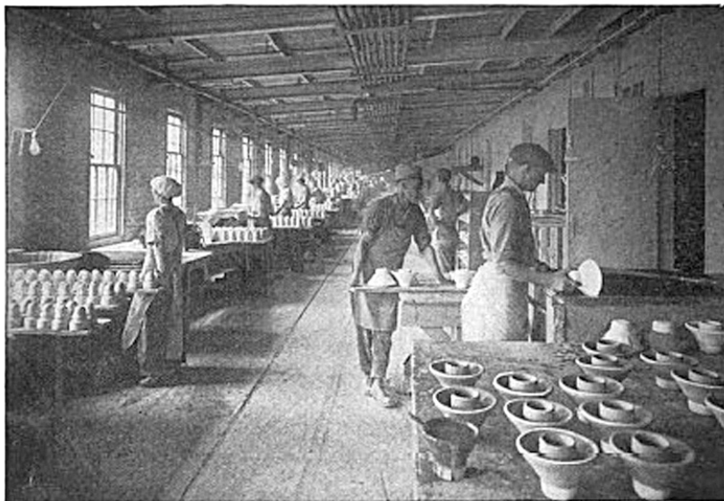
Glazing insulators in a porcelain factory, c. 1920. ( The Clay-Worker , Vol. 73, No. 2, Feb. 1920, p. 148)
