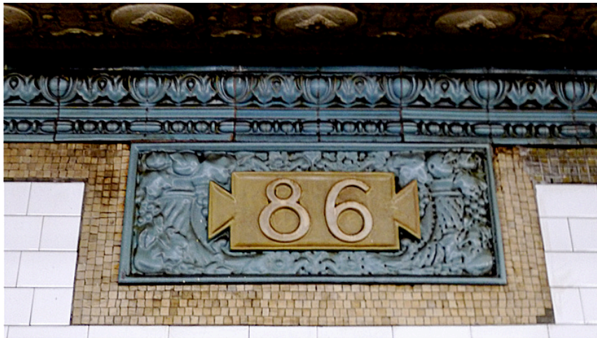
A mass produced, Atlantic Terra Cotta Company cornucopia and street number panel. (Photo courtesy of Michael Padwee)
