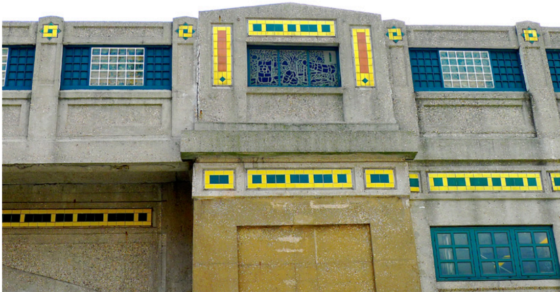
The 33rd Street/Rawson Street/Queens Blvd. station, #7 train
