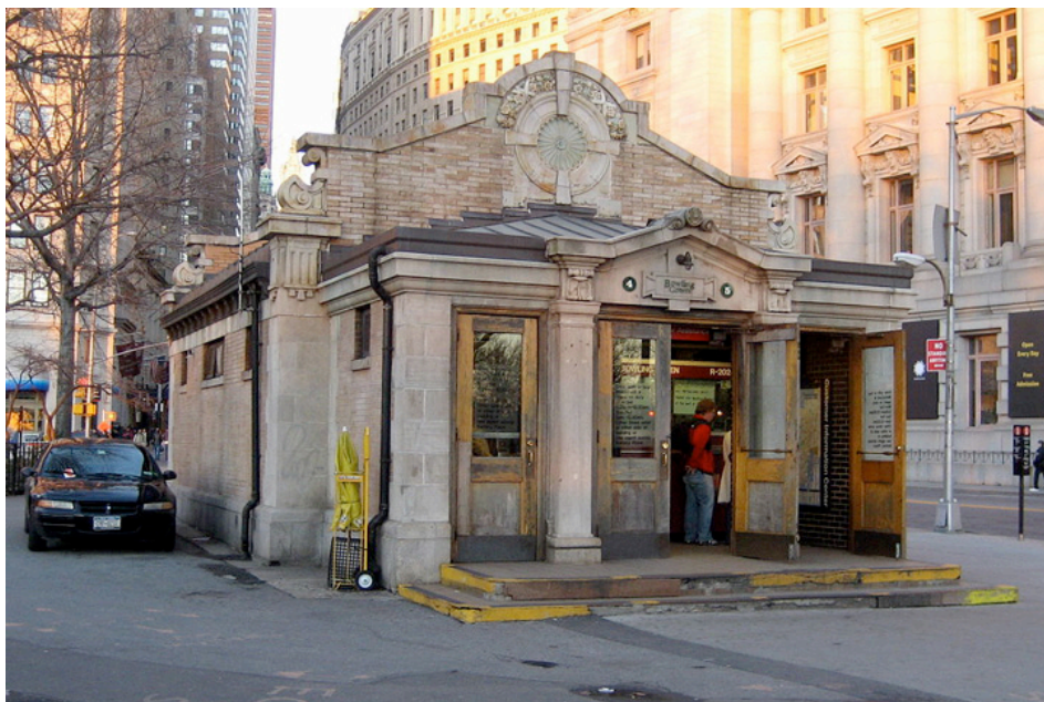
(Photo courtesy of Wally Gobetz ; https://en.wikipedia.org/wiki/File:NYCS_IRT_LexAve_BowlingGreen_ControlHouse.jpg )
