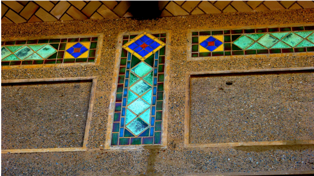
Detail of tiles installed in the station's concrete
