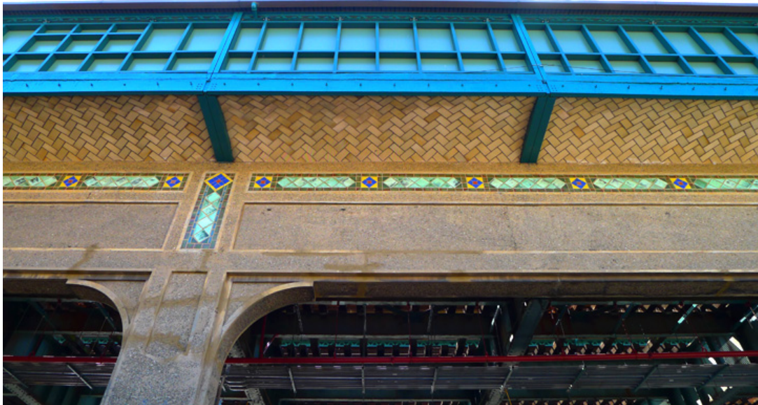
Ft. Hamilton Parkway/New Utrecht Ave. station, "D" and "M" trains
