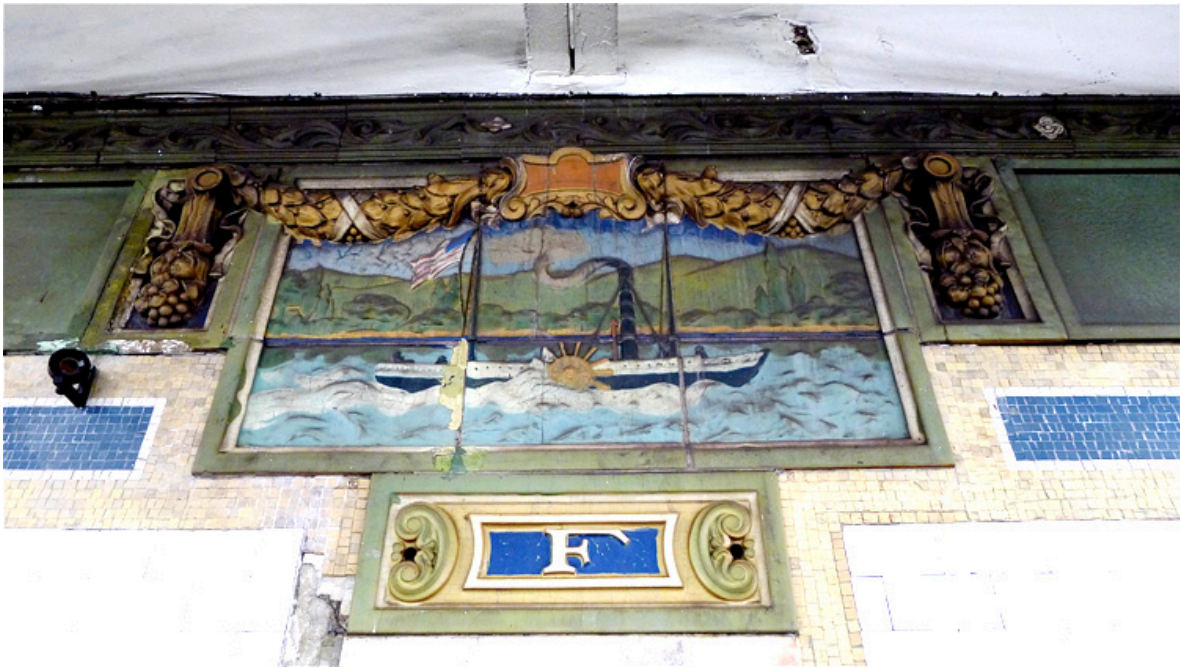
A slightly damaged Rookwood plaque and faience "F" panel at the Fulton Street IRT #6 platform.
