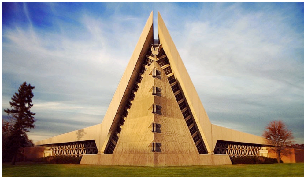
Congregation Shaarey Zedek, Southfield, Michigan (1959-62) was one of Percival Goodman's designs. It rose from flat land and symbolized Mt. Sinai. The 45° dalle de verre windows were designed by Pinart. (Photo from the Shaarey Zedek website; http://www.shaareyzedek.org )
