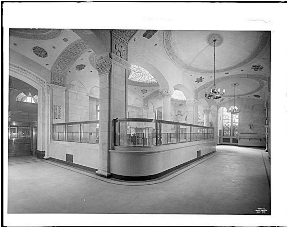
Wurts Bros. (New York, N.Y.) 40th Street and 6th Avenue. Union Dime Savings Bank, interior of officers' section. These three photos are from the Museum of the City of New York Collections.
