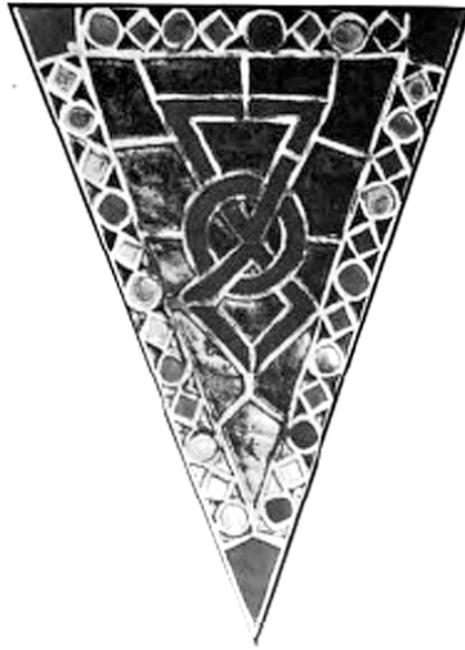
Triangular “Byzantine” pattern made of flat tiles slabbed together in gray cement and ready for insertion in the outer wall of a concrete building 50 feet from the ground. (Mercer, p. 10)
