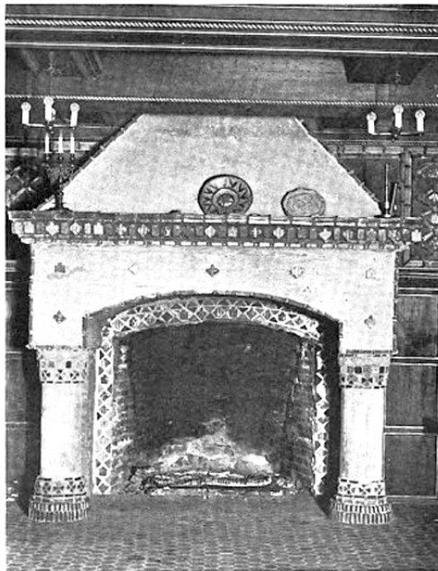
Three views of tiled interior concrete surfaces in the Grill Room and Conservatory of the Raquet Club, Philadelphia, Pa. The tiles are all from Mercer's Moravian Pottery. (Mercer, pp. 17, 18, 20)
