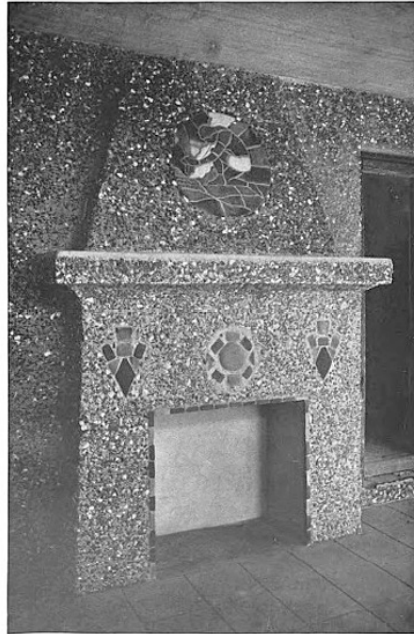
Fireplace on south porch, Mr. Albert Moyer's Residence.
