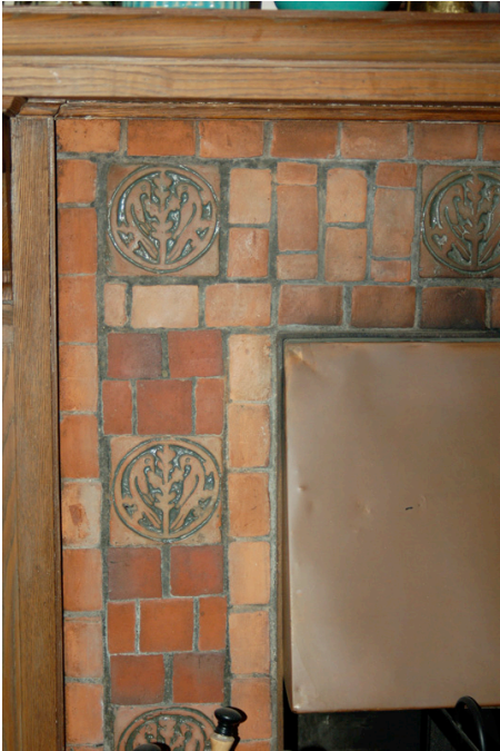
A corner of the living room fireplace with Moravian tiles. (Photos courtesy of Whit Waterbury)
