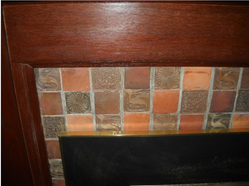
Front hall fireplace detail.
