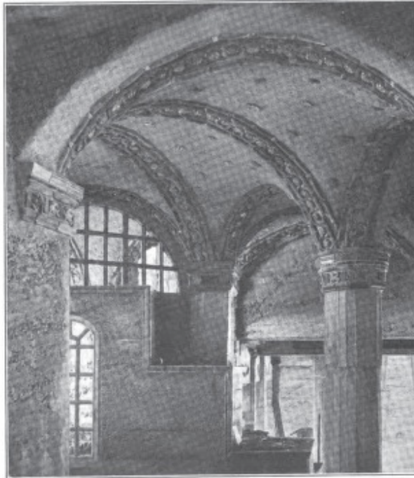
A concrete window sash and tiled, concrete ceiling at Fonthill. (The previous three photos from Frank B. Gilbreth, "Fires: Effects on Building Materials and Permanent Elimination", The Journal of the American Society of Mechanical Engineers , Vol. 83, No. 5, May 1911)
