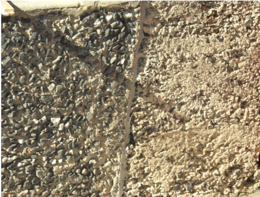
The 2001 concrete aggregate on the left, and the 1906 aggregate on the right, as it looked in 2001. (Photos courtesy of Whit Waterbury)
