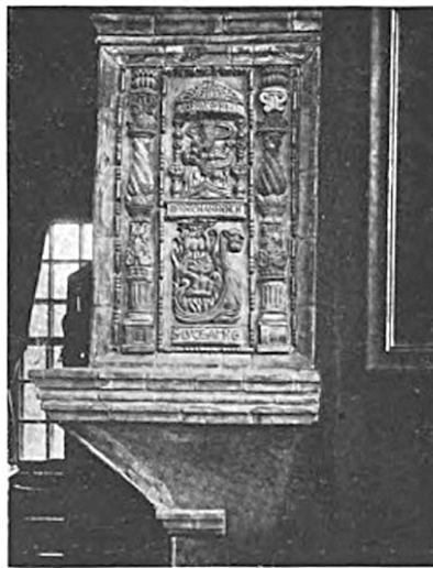
Another of Mr. Mercer's chimney designs that has fine architectural feeling.
