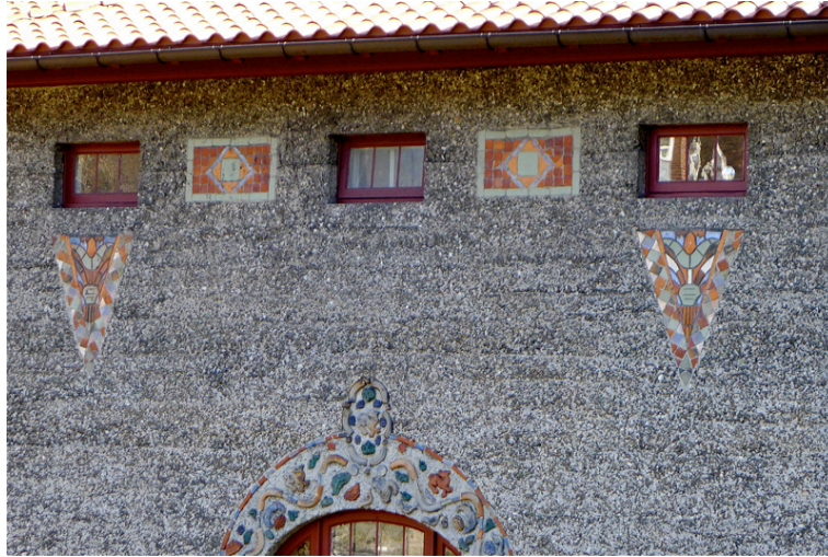
This side of the Moyer house faces the street. The concrete aggregate is broken up by the brightly colored Moravian tile mosaic panels which are above the balcony decorated with Moravian brocade tiles.
