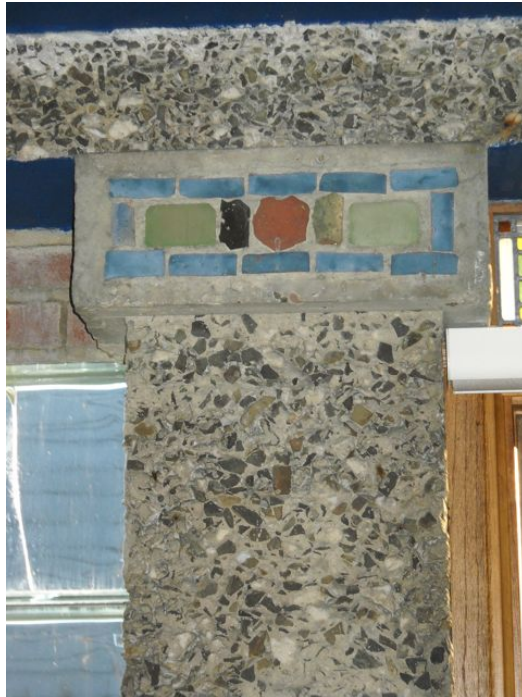
One of six column crowns in the sun room.
