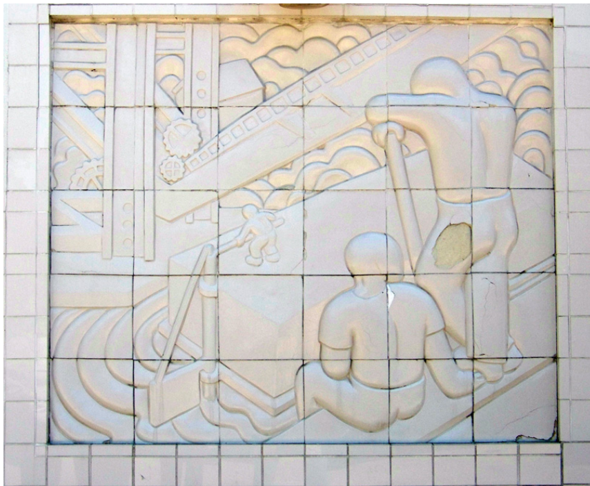
The tiles of the Mortellito Memorial have not fared as well as the original tiles in the WPA murals.
