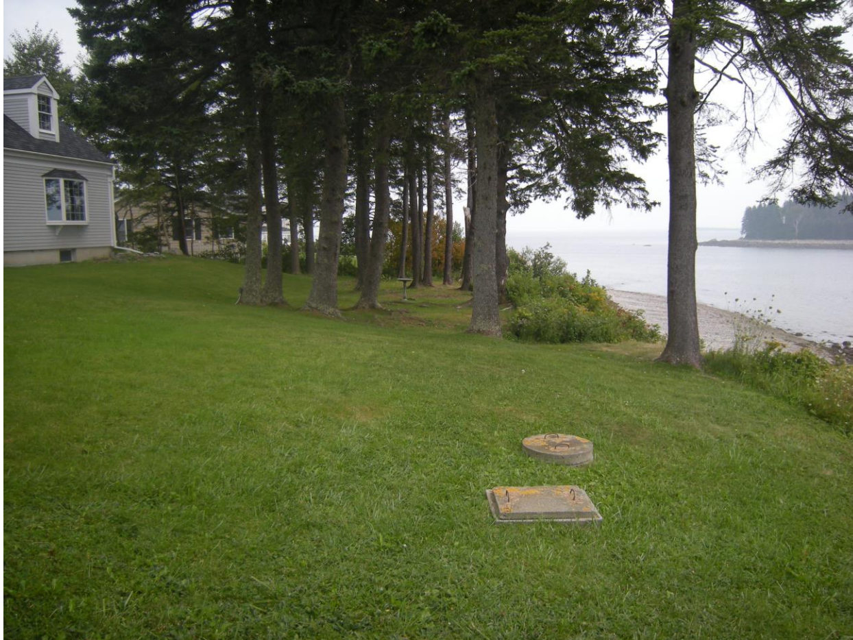
Significant trees and septic system prevent curtain drainage Owl's Head
