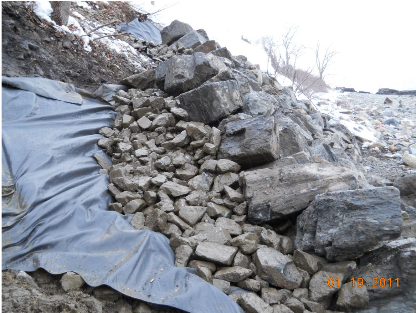
Armor layer showing riprap underlayer and geotextile. Lincolnville
