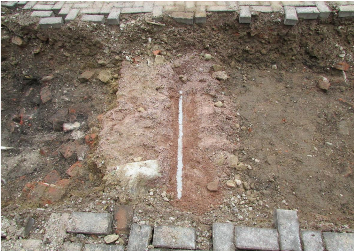
Figure 22. Modern BT service in trench 5. To left (017). To right (019)
