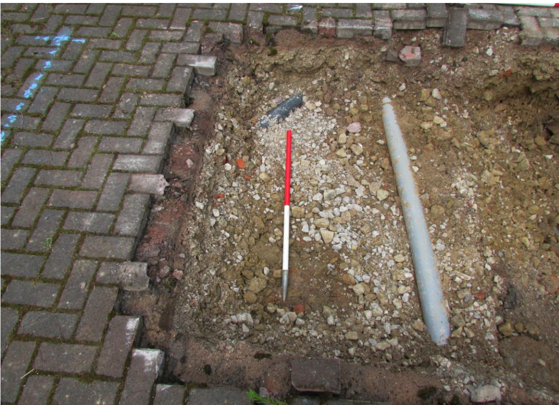
below Figure 38. Shot of modern services running through the south-west of trench 6.
