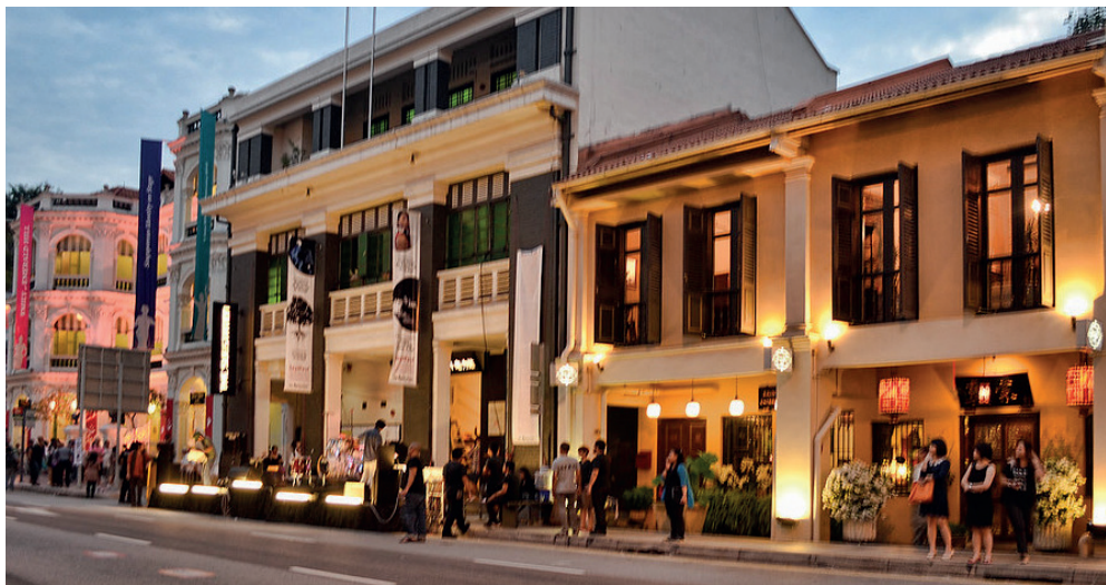
The Substation, image by Choo Yut Shing, 2012 www.flickr.com/photos/25802865@N08/7933525394 , some rights reserved
