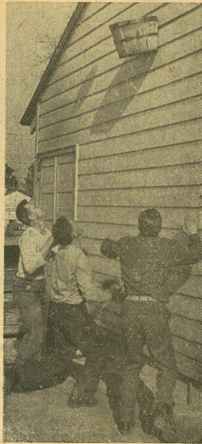
Before our carpenters went to work.
