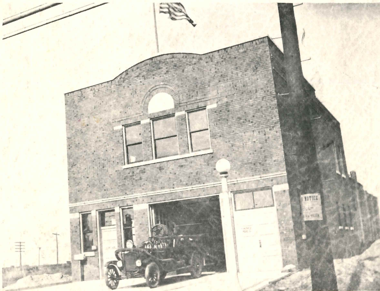
Village Hall Building, 1927. Take note of the fire fighting apparatus.
