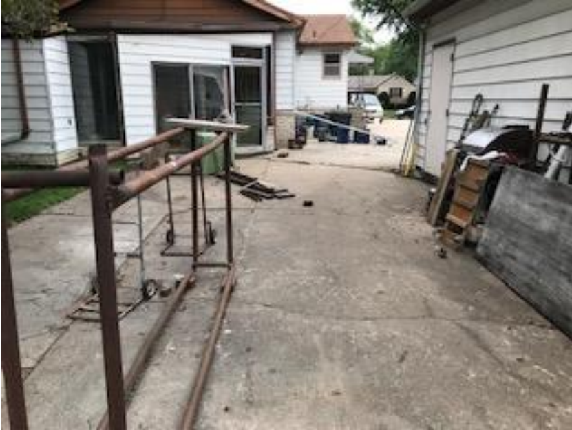
Before view from the back. On the right is the west side of the huge garage. At left in foreground is one of three metal firewood holders left by the previous owner.
