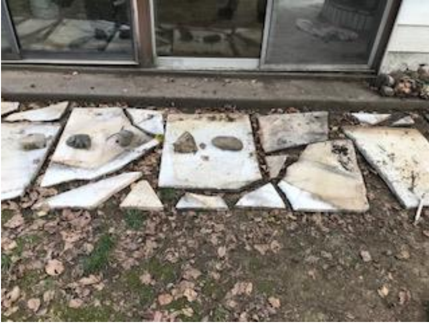
Small patio in process.
