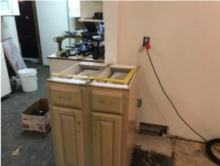
Kitchen in process
