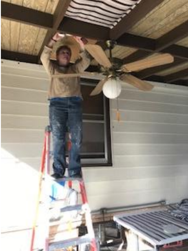
Sarah putting fabric on the porch ceiling. The original "paneling" was paper which disintegrated when painted. The necktie fabric was left over from another project. There was just exactly enough! The fabric covered lots of unsightly nail ends which could not be cut off.
