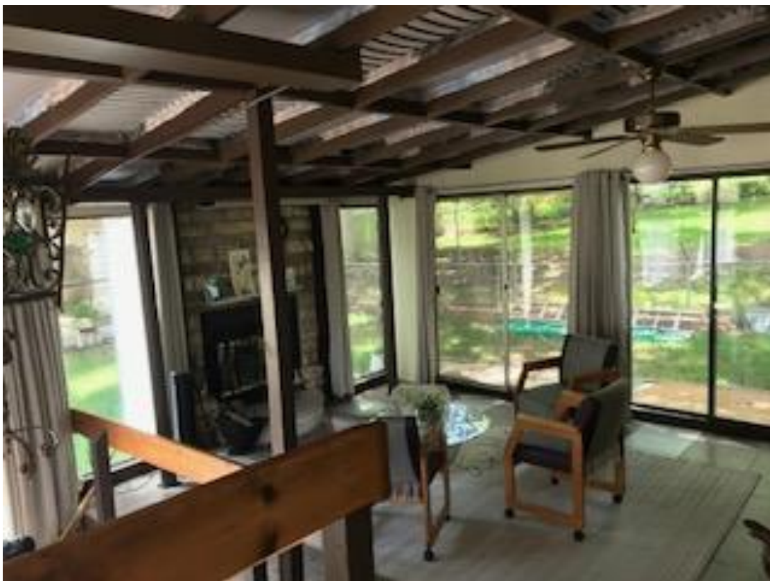
After: Five of the door-sized windows and two of the screens on the closed-in porch were replaced. The shag green carpet was torn up and Dan tiled the entire area, steps to the basement and all.
