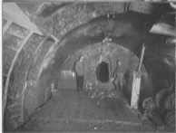
HOSPITAL AIR LOCK, where walkmen are tested for the "bends" in reduced pressure. FIRST PASSAGE UNDER HUDSON RIVER, north side of Hudson & Manhattan tunnels from Morris St., Manhattan, to 124th St., J. C., Sept. 29, 1875; begun 1872; twice abandoned.
