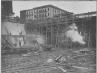
EXCAVATING under 4th Ave. "L" for cut through which materials from station excavation are carried to mows which are towed to Greenville, N. J., to fill in great freight yard. EIGHTH AVENUE, with trolley line supported on trestle during work on station excavation.
