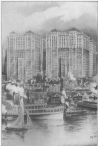
CHURCH ST. TERMINAL , largest and heaviest building in city; 200,000 tons, including 24,000 tons structural steel, 17,000 tons concrete, 16,500,000 bricks, 4,000 tons terra cotta, 188,000 sq. ft. glass, 120 miles of pipe, 17 1/2 miles wiring, 50 electric elevators, 28 stairs, 27 1/2 ft. above city water structure, 18,150,000 cubic ft. Clinton & Russell, Architects.
