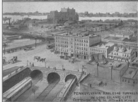
POWER HOUSE , Long Island City, 4,000,000 ft. with coal tower 170 ft. high; 24 5,000-horsepower generating units; 28 tubular boilers; George Gibbs, chief engineer electric traction. LONG ISLAND CITY , emergence of tunnels and connection with Long Island RR. system.
