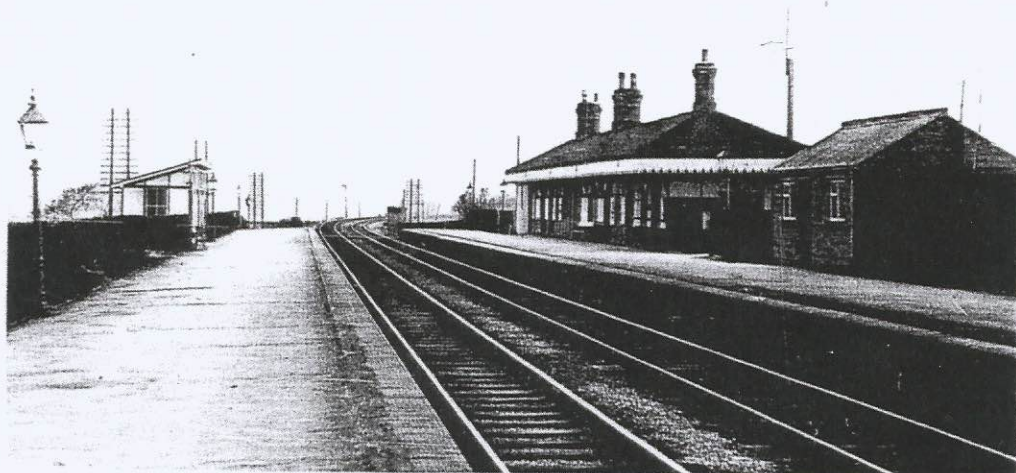
Old Dalby station looking North 1955
