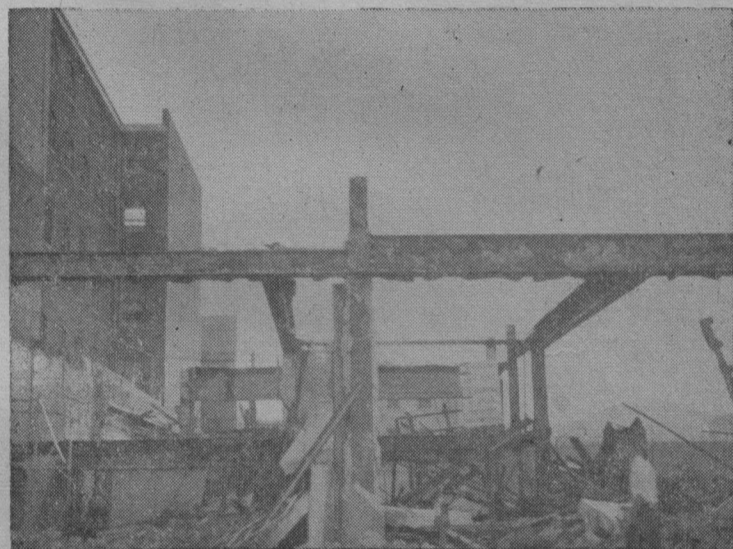
Site being cleared for new building.
