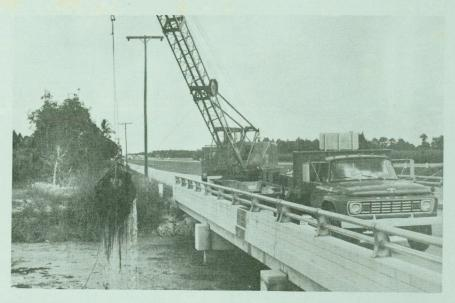
BIG JOB of aquatic weed control sometimes takes big equipment such as this dragline and truck. A steel A-frame attached to a boat tore underwater weeds loose so they could float to the 'pick-up' point.
