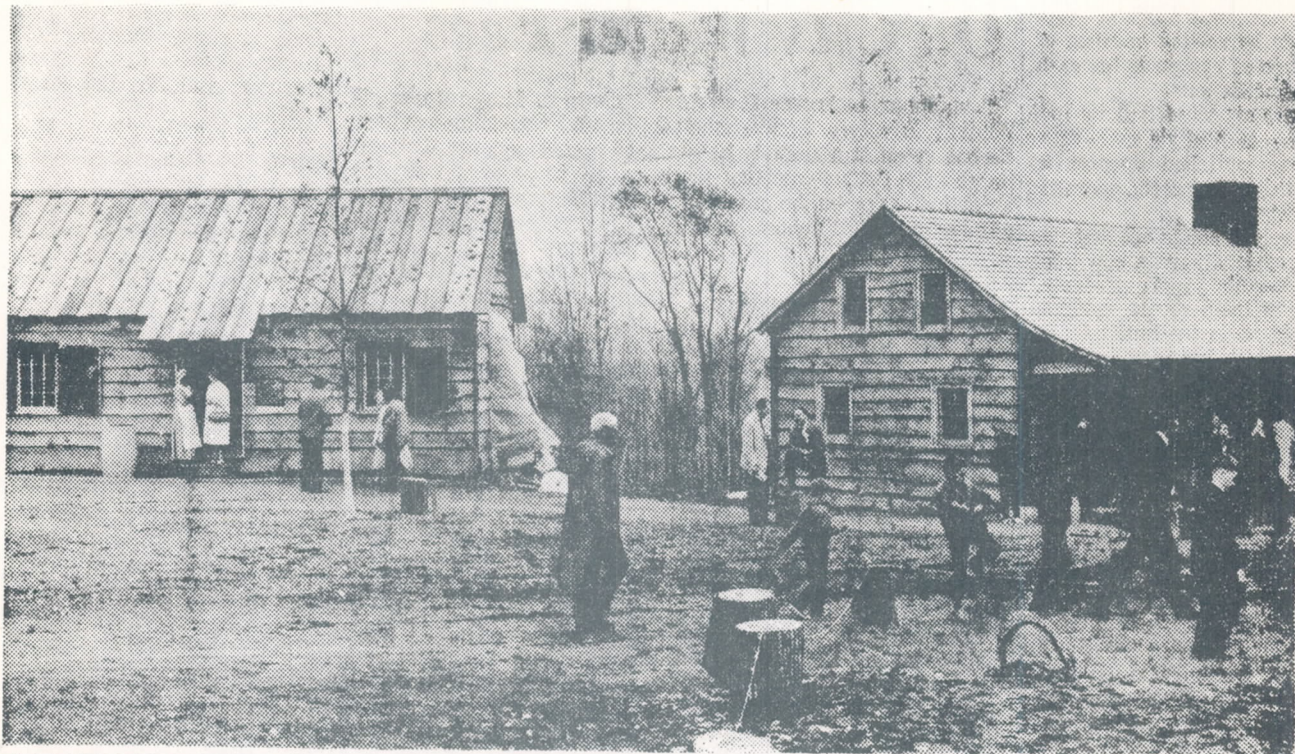
10 BUILDINGS IN ALL — Two of the newest buildings at the cantonment are the Armorers Shop
