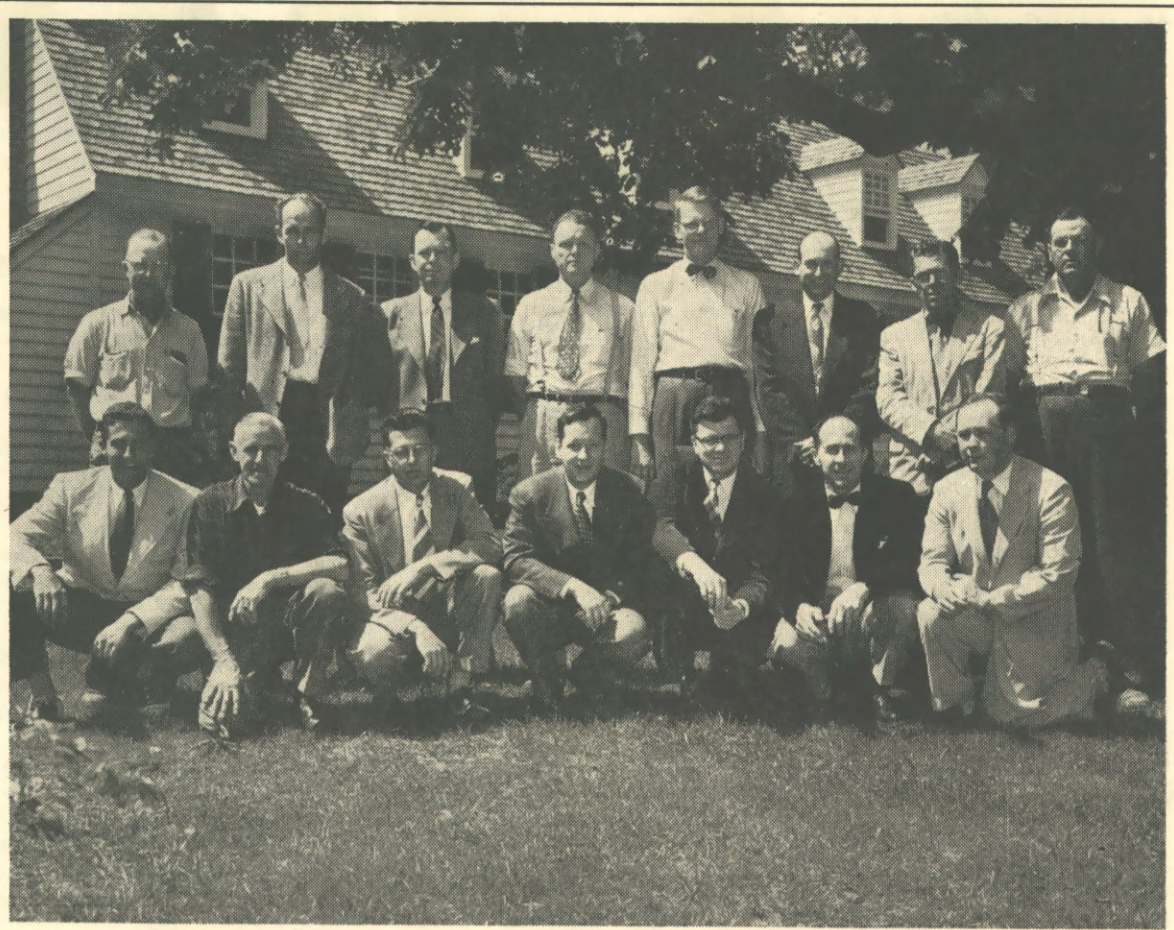
AT WALLER HOUSE this group of architects, landscape and construction supervisors, all of whom worked on the restoration job, pose for a record photograph. They are (kneeling, l. to r.) Dick Mahone, Bill Keller, Ernie Frank, Tom Drewry, Don Parker, Leroy Phillips, Paul Buchanan; (standing, l. to r.) Arthur Wilson, Alden Eaton, Alden Hopkins, "Red" Vaughan, Roy Tait, Milton Beverly, Lyman Peters, and Bruce Hardy.
