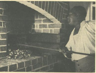
THOROUGHLY FIRED, an oven is made ready for baking by Baker's Assistant Victor Valentine, who rakes it clean of wood ashes. The red brick oven is dome-shaped, has walls 18 inches thick and is set in two feet of solid brick. It is built on original foundations.
