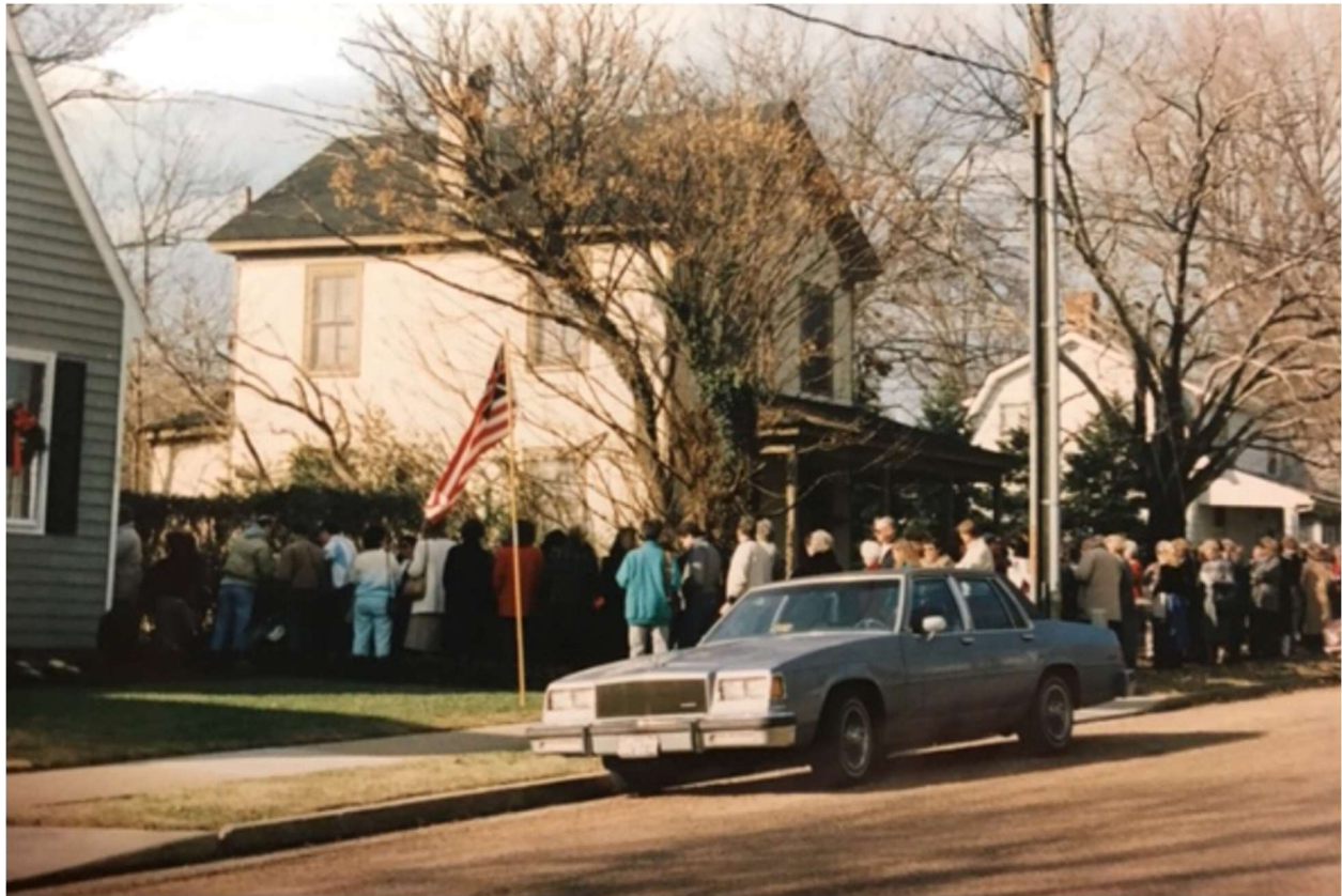
Figure 6: Photo of Jerome Casey House (Block 45, Building 27) prior to demolition. Image courtesy of Bo Parrish.
