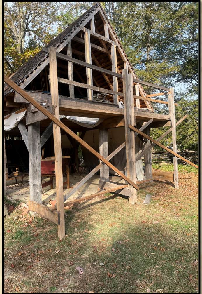
Scaffold to access the gable end door.
