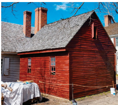
The Anderson Armory Kitchen with a new coat of red pigmented tar as it appeared in winter 2019.
