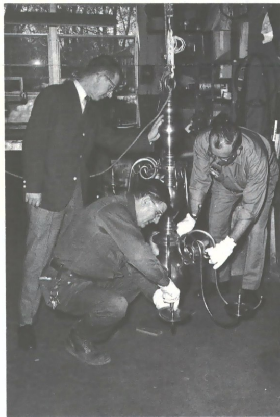
Royce Cottingham, director of Mechanical Operations and Maintenance, watches as Robert Eheart and James Jenkins, maintenance servicemen in MO&M, assemble an 18th century chandelier before electrifying and hanging it in the Chapel of the Christopher Wren Building at the College of William and Mary. The chandelier is made of hand casted brass and weighs nearly 400 pounds.
