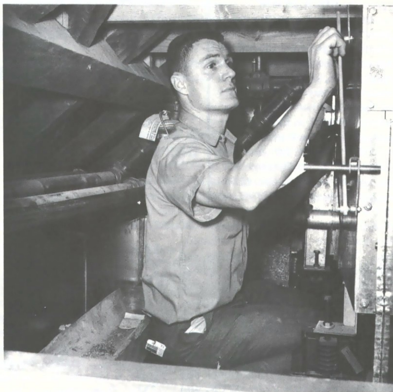
Armond Campbell, sheetmetal worker in the Department of Mechanical Operations and Maintenance, adjusts damper linkage on one of the air handling units now installed in the attic of the Peyton Randolph House, an exhibition building that will be opened to the public this summer.
