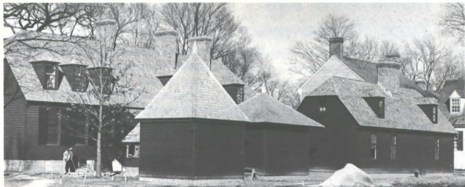
A view of the Wetherburn Tavern outbuildings which are scheduled for completion by February 15.
