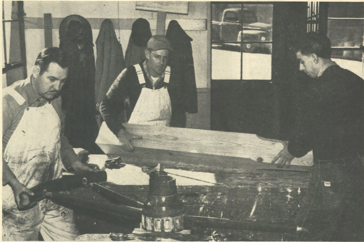
ALL IN A DAY'S WORK , these carpenters busy themselves with some of the routine projects handled at the warehouse shop. Arthur Ward (left) adjusts section of rim to spokes of one of the 18th century carriage wheels being repaired, while R. E. Holland (center) and George Temple do some of the preliminary shaping on one of the fence posts constructed for the Restored Area.
